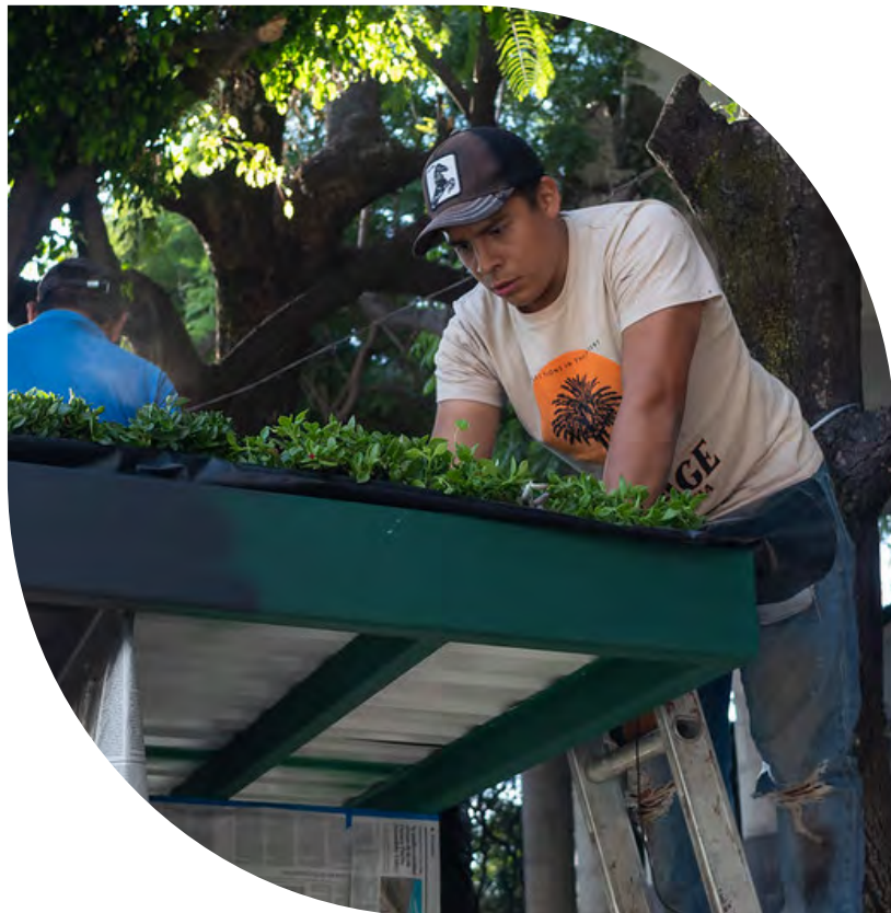
Both images: Installation of a green-roofed bus stop on the 16 de Septiembre Avenue, August 2023. © WRI México
